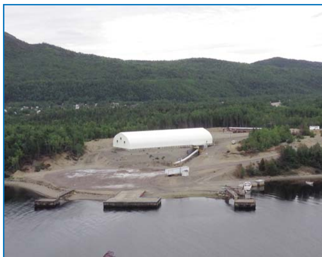
Rambler's concentrate storage shed at Goodyear's Cove
